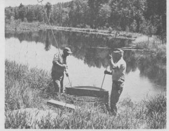
Removing stop logs on the water control structure of a multipurpose fish and wildlife pond.
