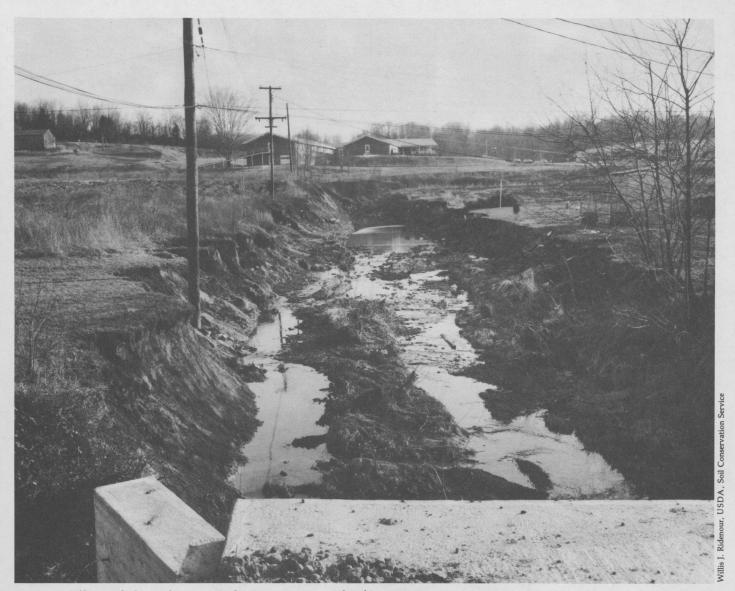
Figure 6. Effects of channelization and improper stream bank protection.
