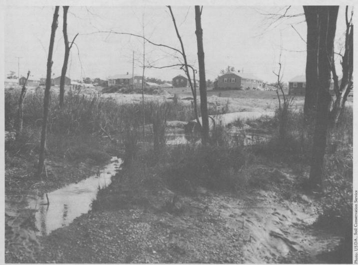
Figure 36. This storm sewer outlet, emptying only 50 or 60 feet in back of a stream, causes ponding and health hazards.
