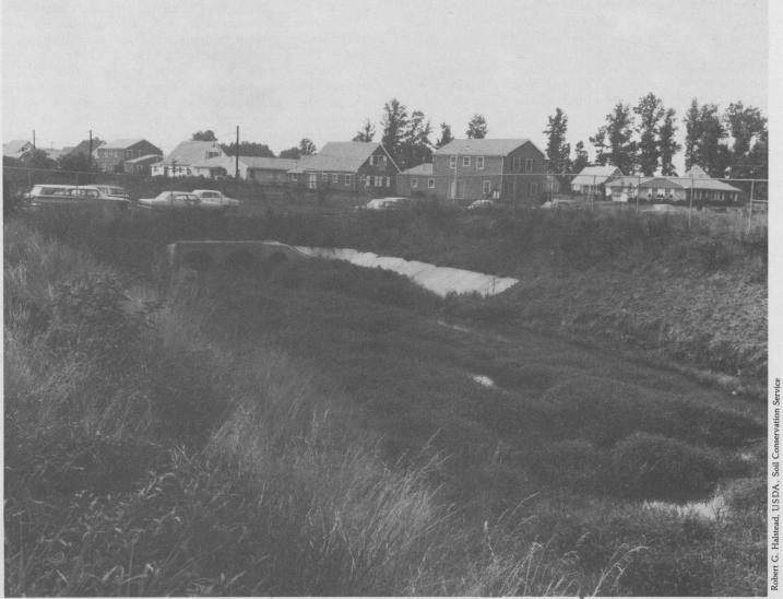
Figure 4. Sediment deposits from development construction have almost completely filled in and blocked up this ditch.
