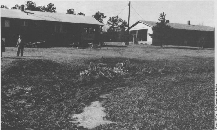
Figure 35. This is ponded sewage effluent from a septic field on soil with severe limitations for such use. It has a disagreeable odor, and it is a sanitation hazard. When tile lines are punched with a probe, the effluent rises to the surface.
