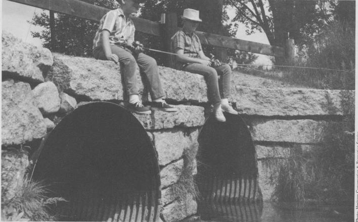
Figure 33. Culverts should be designed large enough to permit fish passage.
